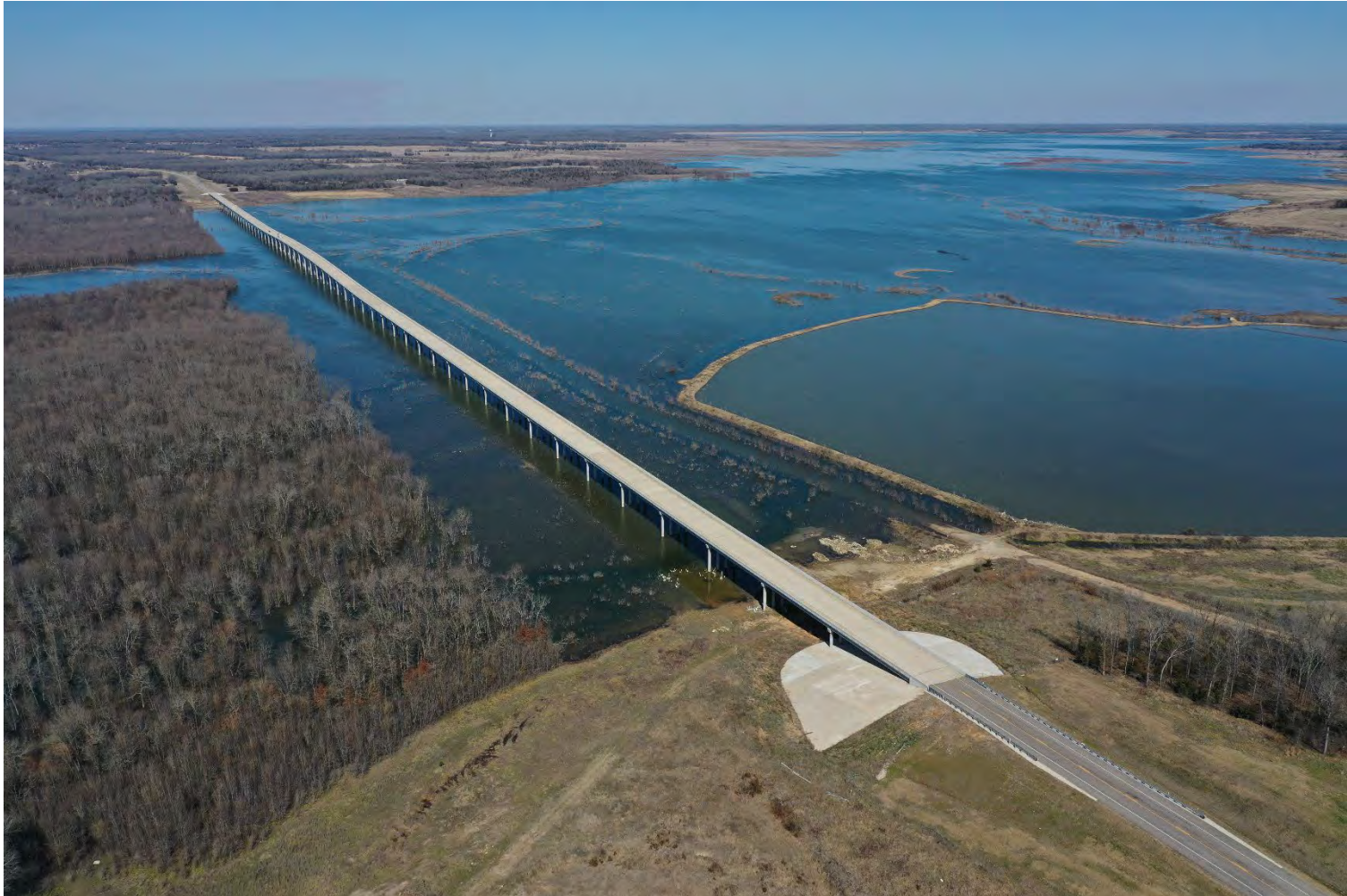
FM 897 Bridge Complete and Open
