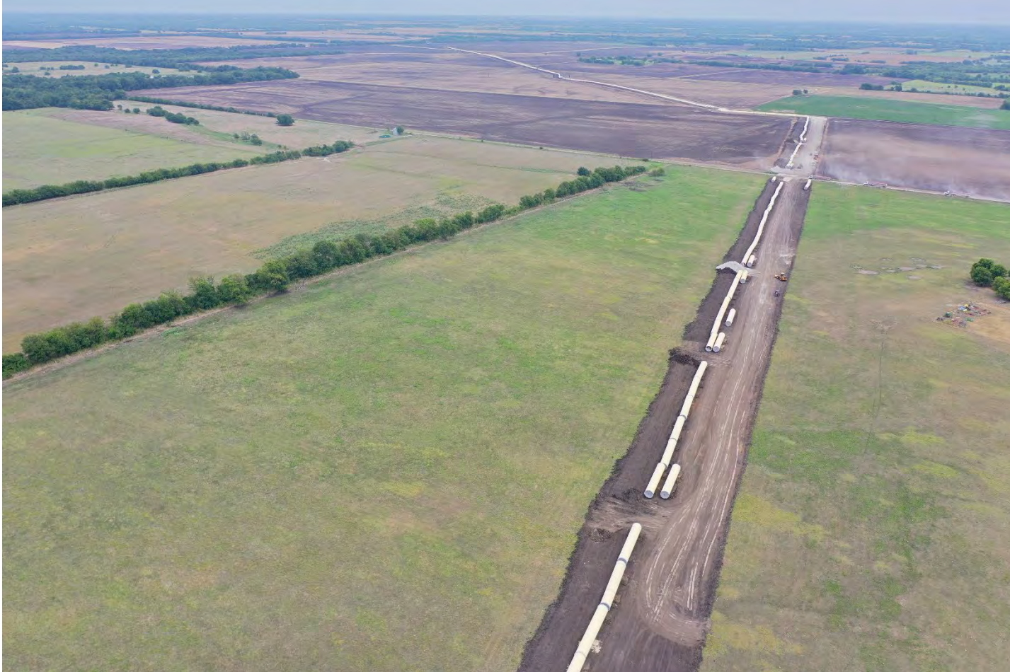
Raw Water Pipeline Installation
