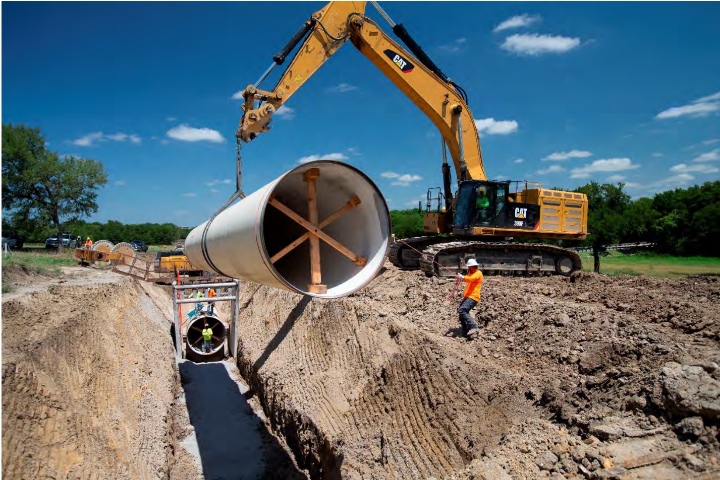
Treated Water Pipeline Installation
