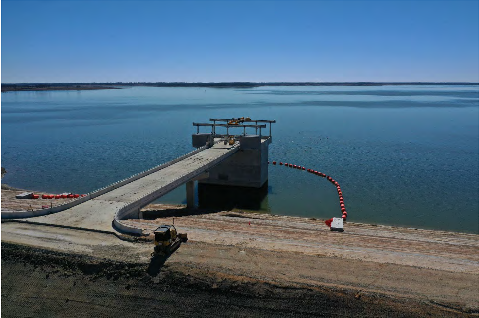
Intake Tower Construction and Wet Side Impoundment
