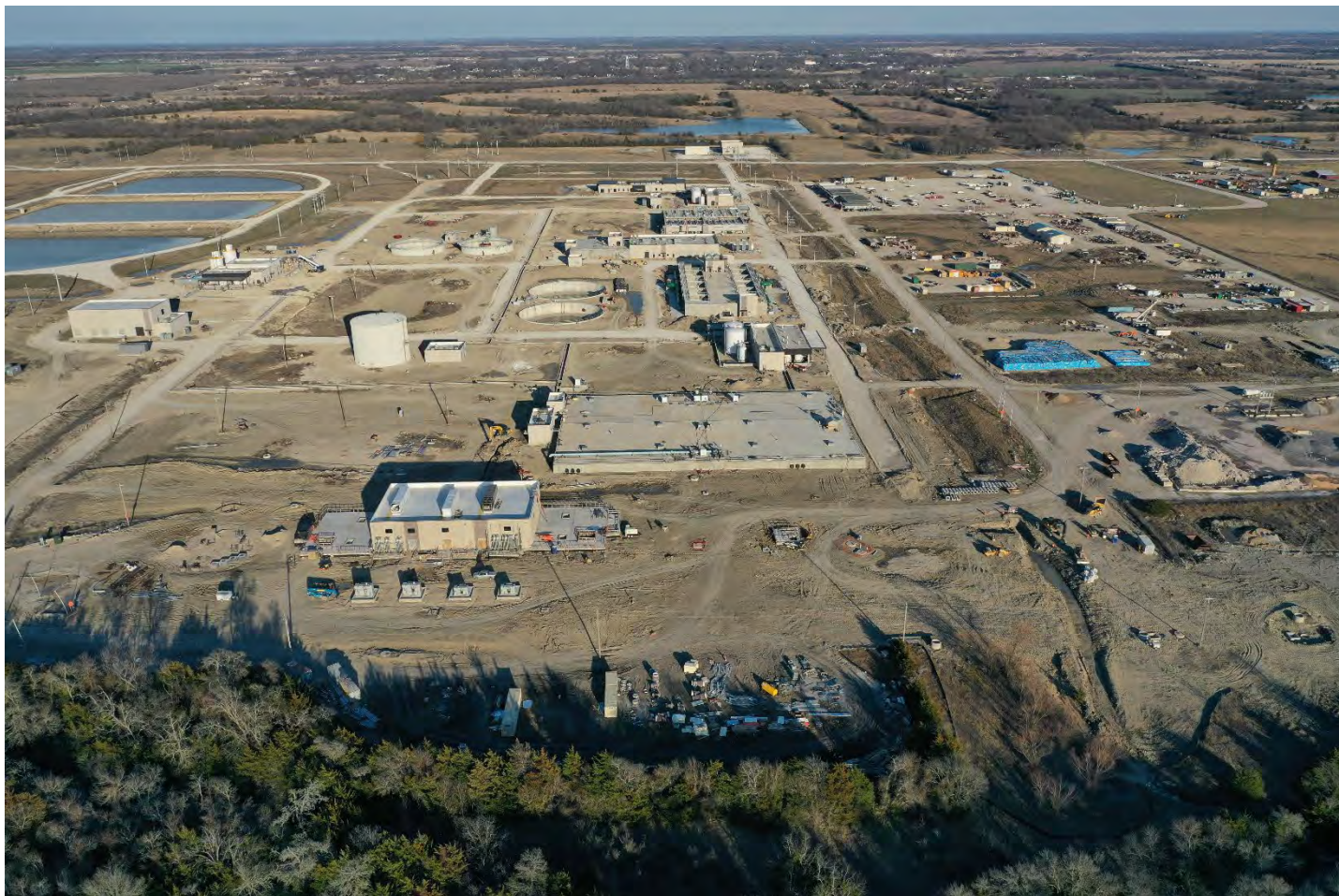
Leonard Water Treatment Plant
